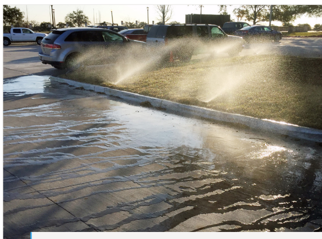
Figure 1. Example of runoff from spray head sprinklers.
